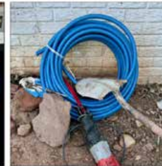
Figure 9.2 Sharp Objects Can Damage PEX
